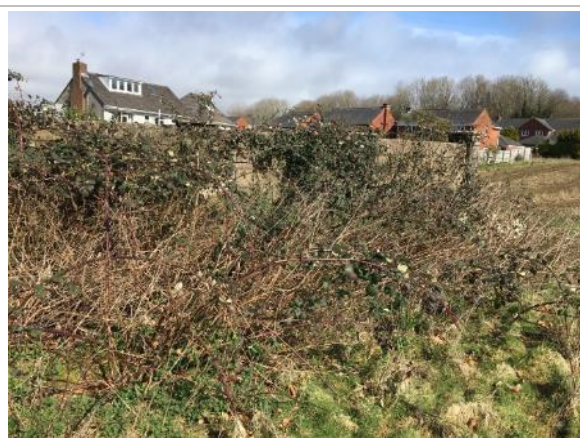
Photograph 3: Dense bramble scrub south of the cinder block wall located in the northwest of the Site.
