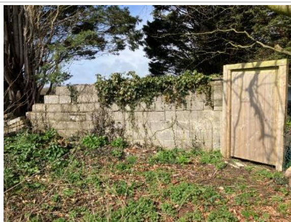
Photograph 16: Cinder block wall in northwest corner.
