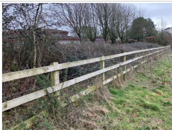
Photograph 15: Wooden fence with wire on eastern boundary.
